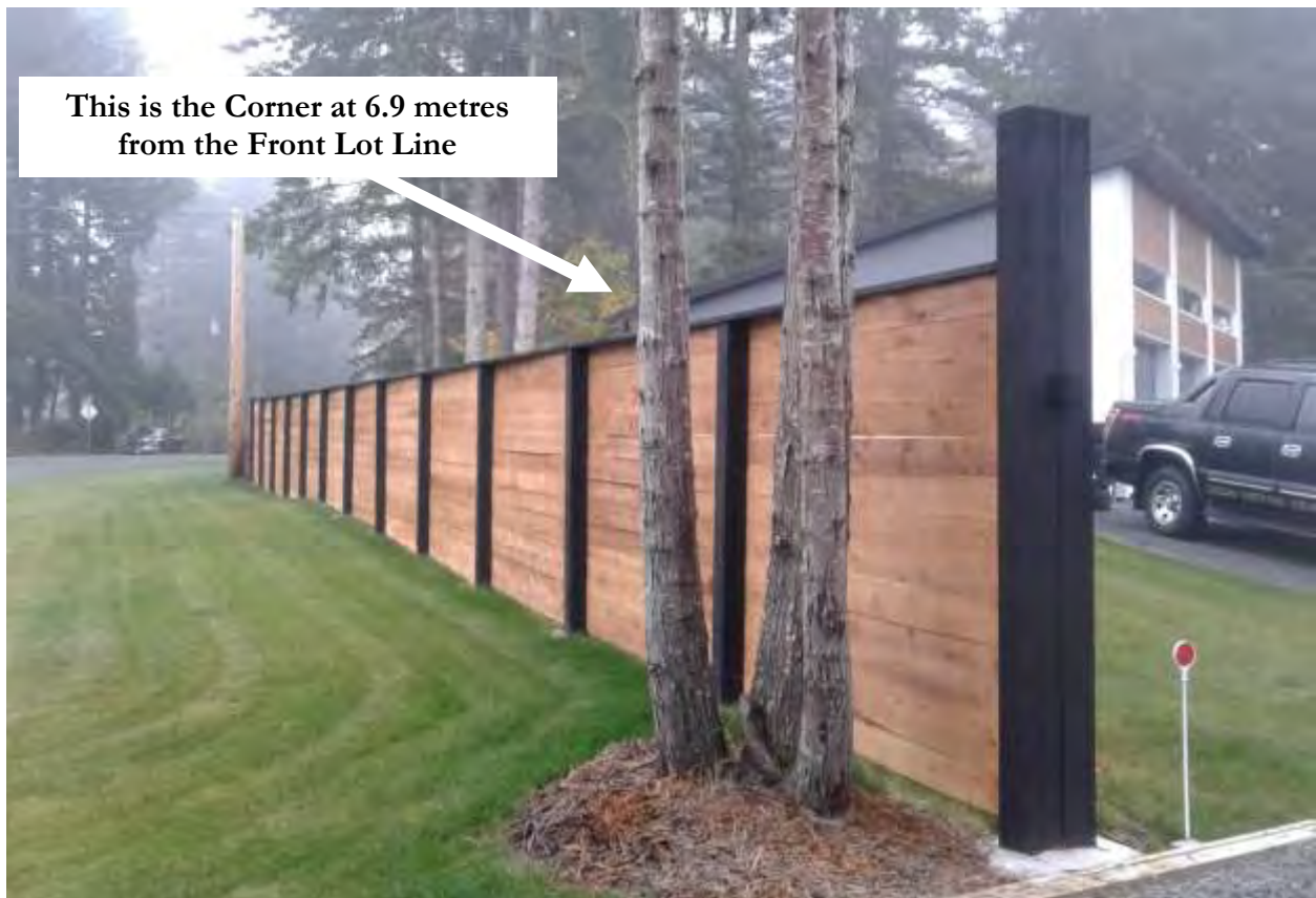
Figure 5: View of the Accessory Building from the Driveway
